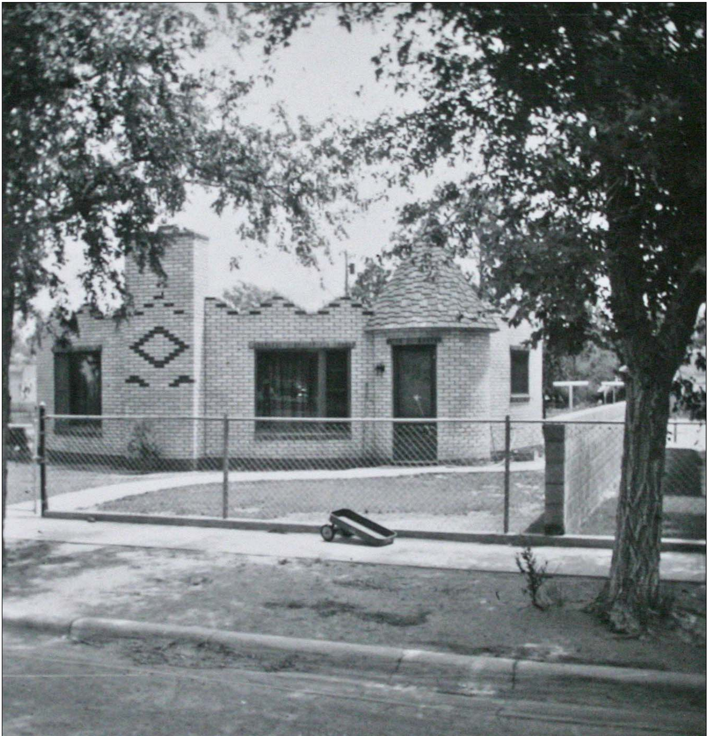
Figure 2. This Kiowa County Assessor appraisal card photograph shows the house in 1955. The house then featured: front windows with a picture window and a four-part casement window; a wood slab door with three stepped, rectangular lights; and decorative wood shingling on the conical roof of the entrance. A clothesline is present in the southeast portion of the parcel; the sheds and pavilion are not present. Courtesy of Kiowa County Assessor, Eads, Colorado.
